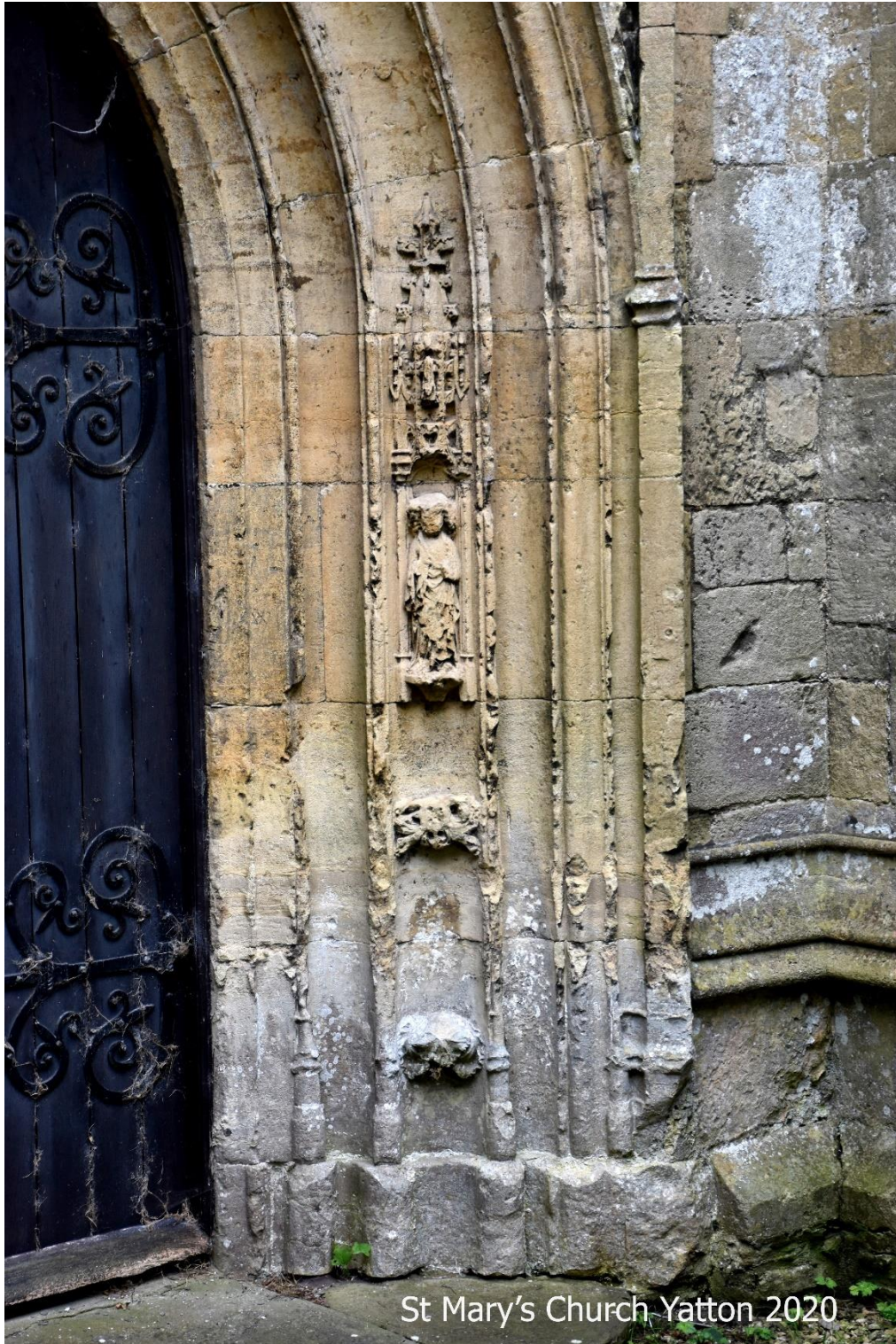
Fig 56: Right hand side of doorway.
