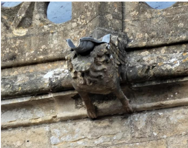
Fig 17: Below upper parapet. Left hand side
