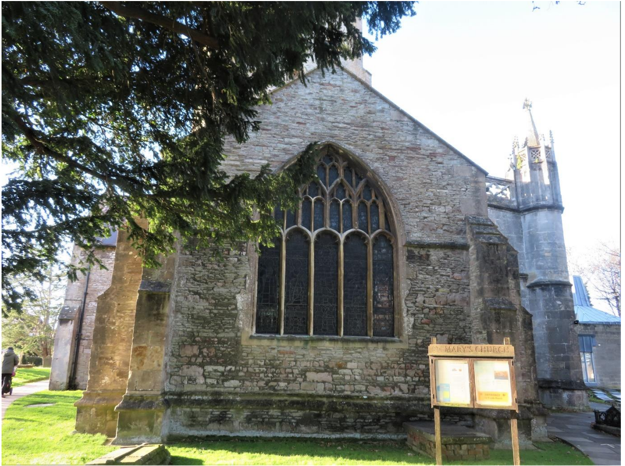
Fig 78: The east end of the church.
