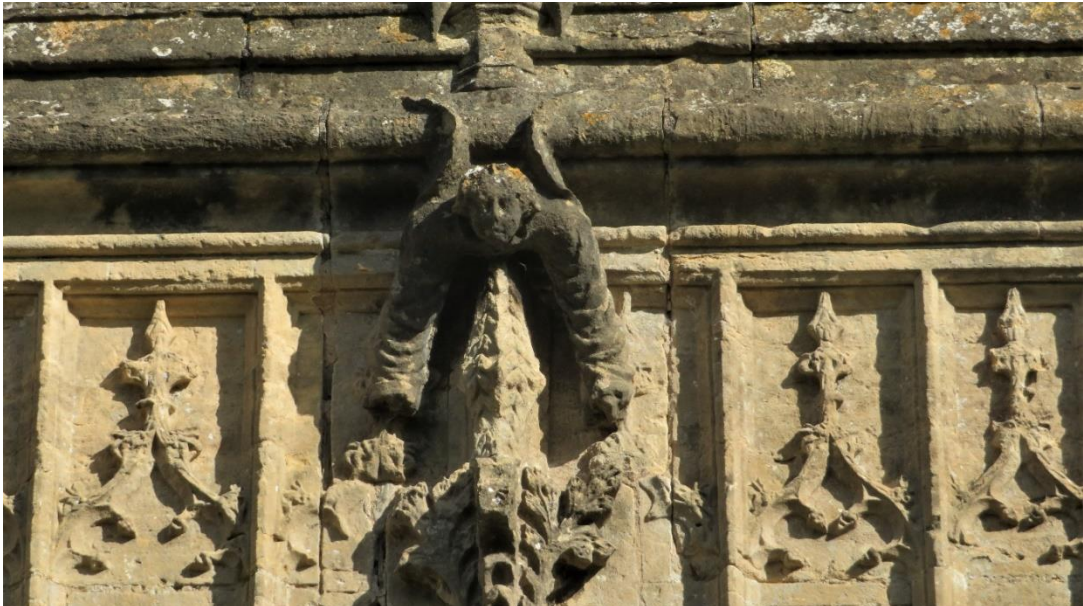
Fig 25: An angel under the parapet.
