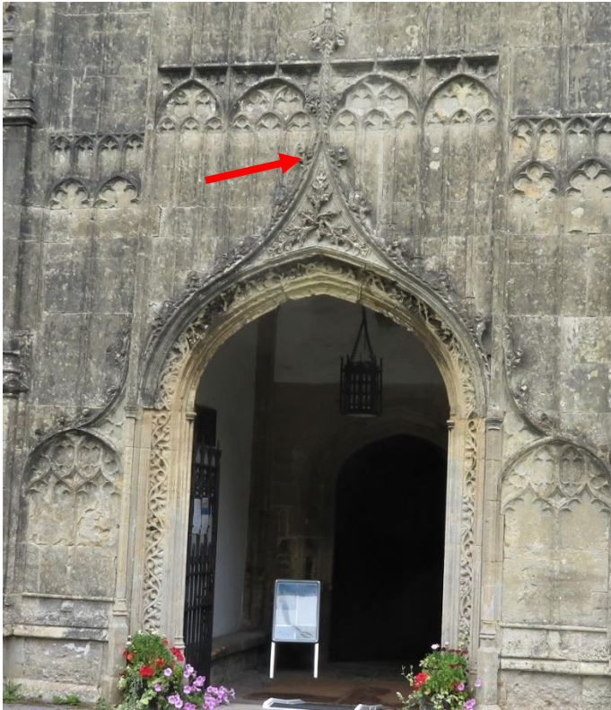
Fig 20: Close up of doorway.
