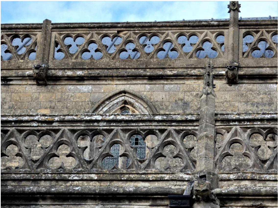
Fig 15: Close up view of parapets right of the south porch.
