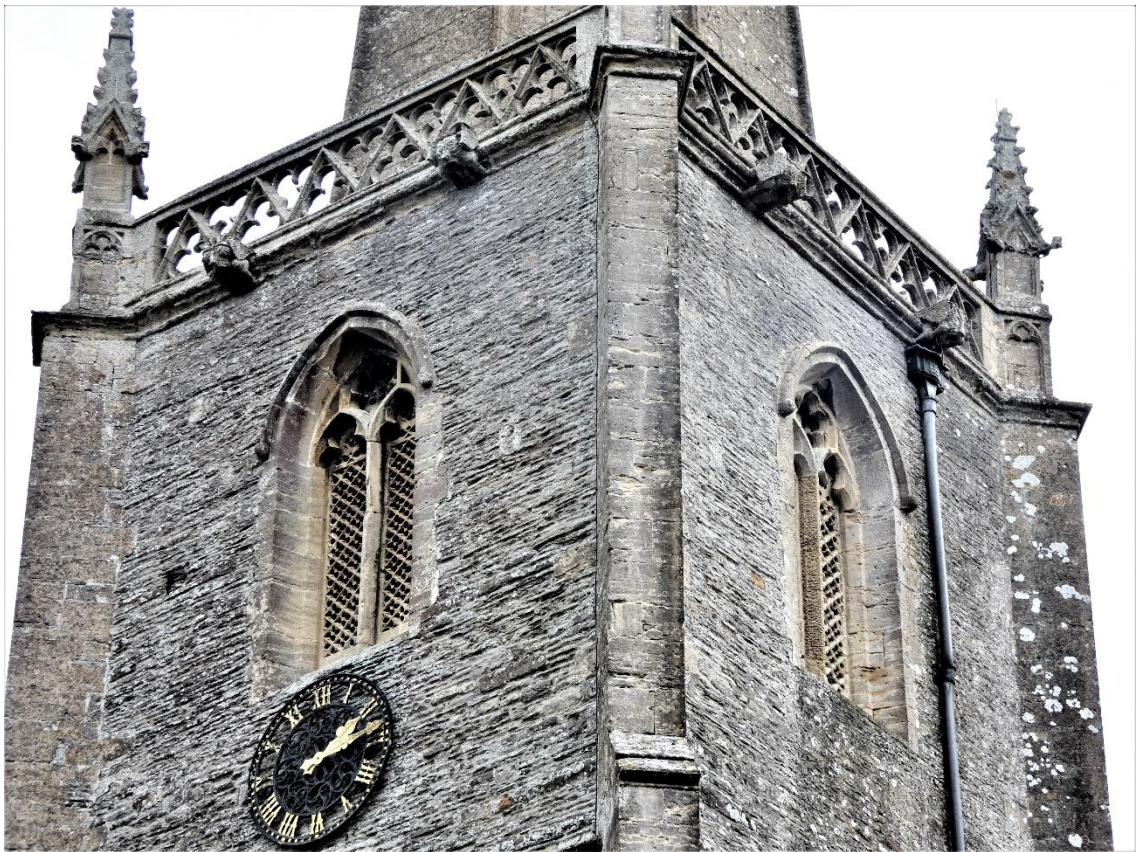
Fig 82: The north side of the tower with the clock face.
