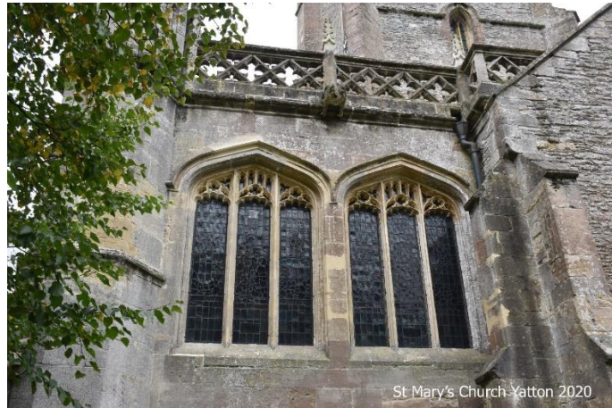
Fig 76: A view of the parapet.
