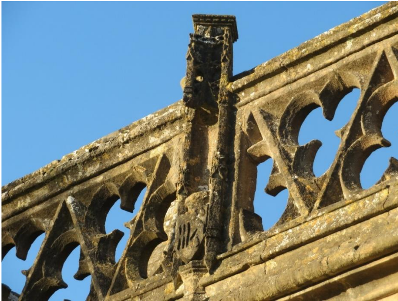
Fig 23: Parapet above porch.
