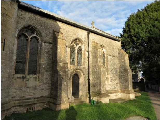
Fig 5: East end showing doorway.
