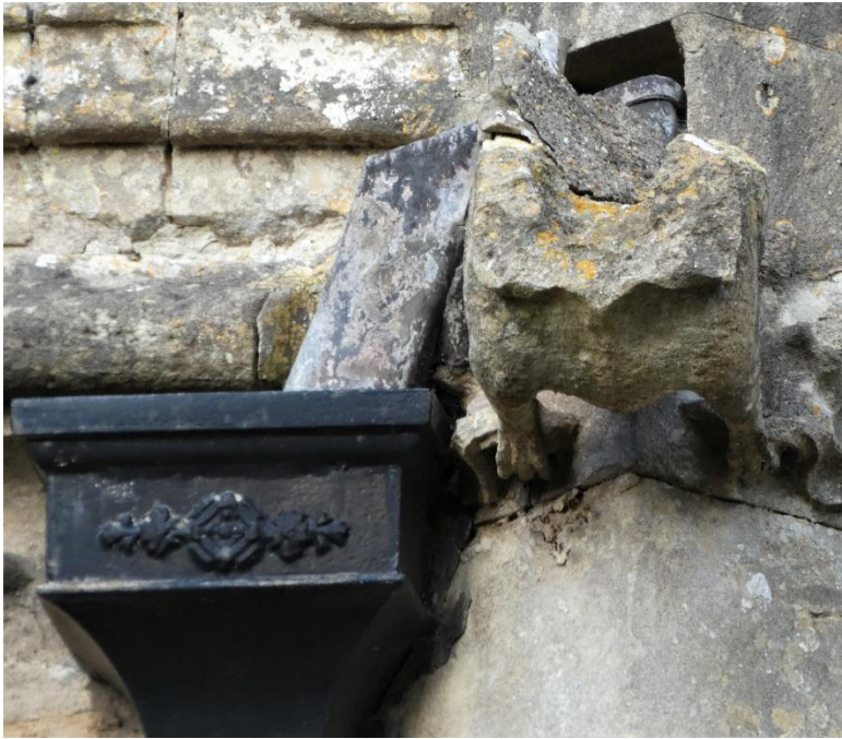
Fig 16: Below bottom parapet
