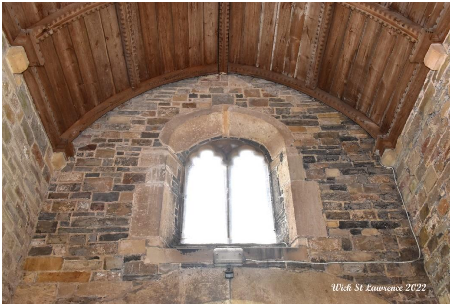
The south window of the porch.
