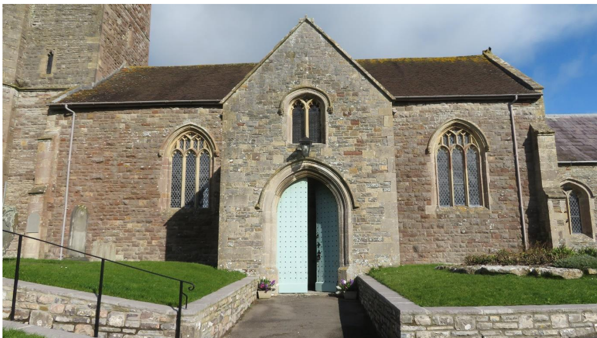
The porch was rebuilt in 1865.
