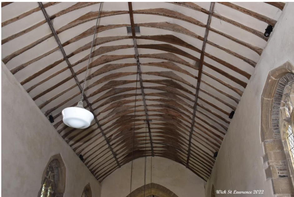
The nave roof.
