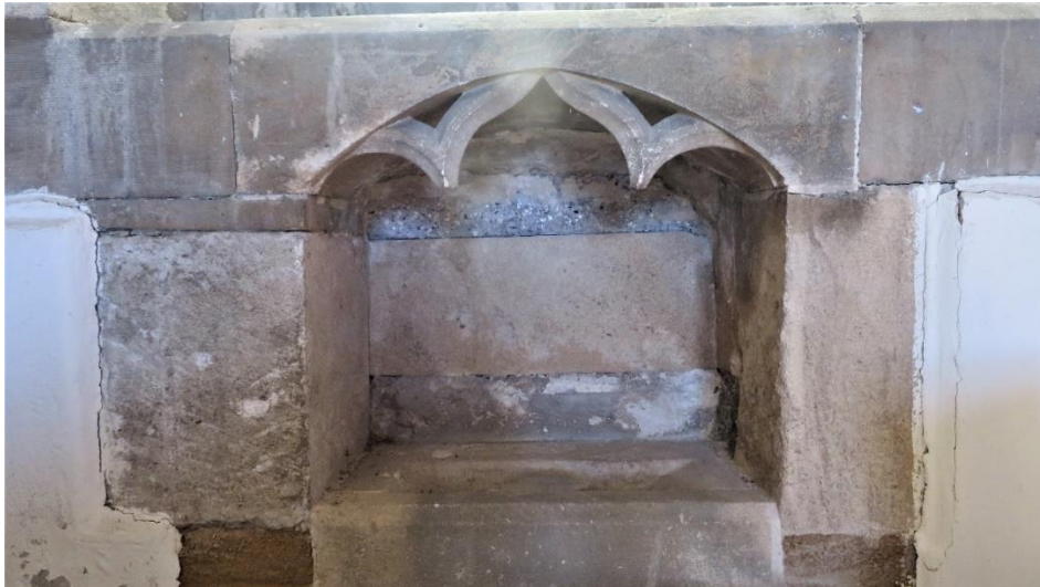
Below the window is this piscina which was used to wash the vessels after mass. Little of the original work remains.
