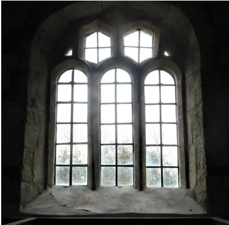
South side by plaque / east of blocked door. This three - light window is probably 17th century in date.
