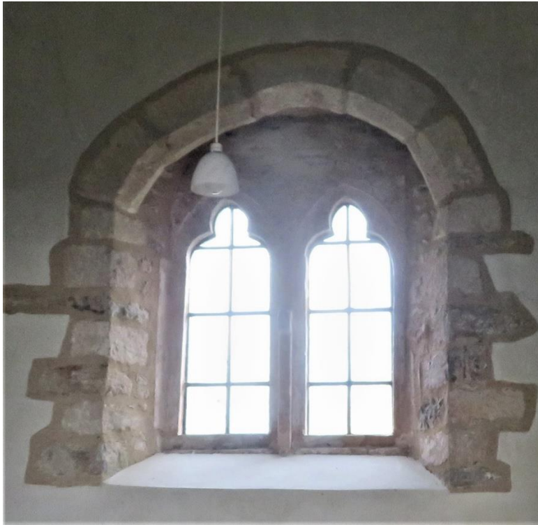
North side west of door. This very small two-light window has sharply pointed trefoil heads on each light and may date to the 14 th century or even late 13 th century.
