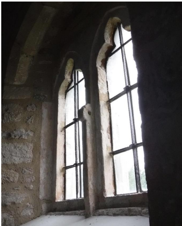
This window also has shutter rebates and a bolt socket.
