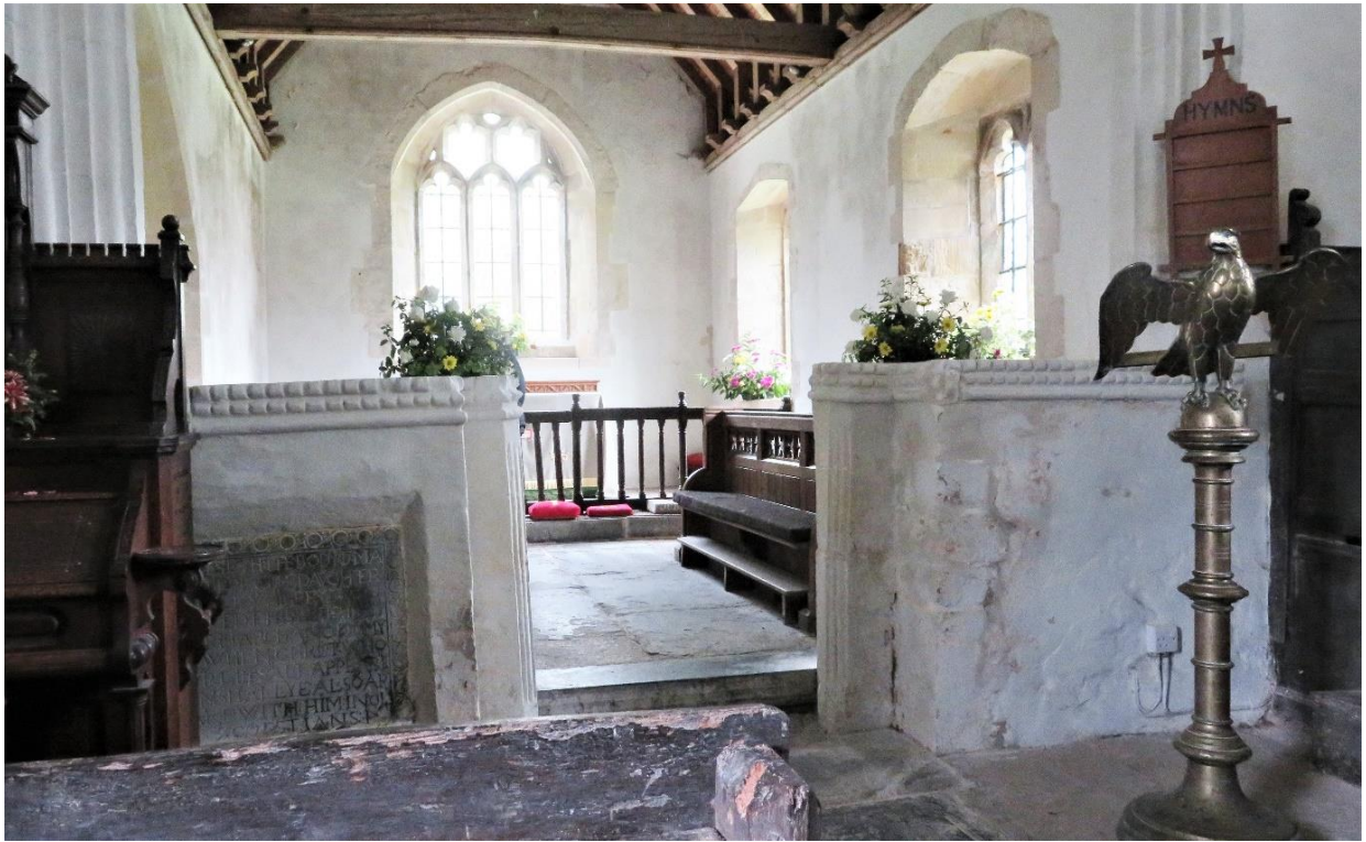
The stone chancel screen, plainly cut into the chancel arch, survives to waist height. It is thought to be 16 th century and may have formed the base of the rood screen or replaced the rood screen after the Reformation.
