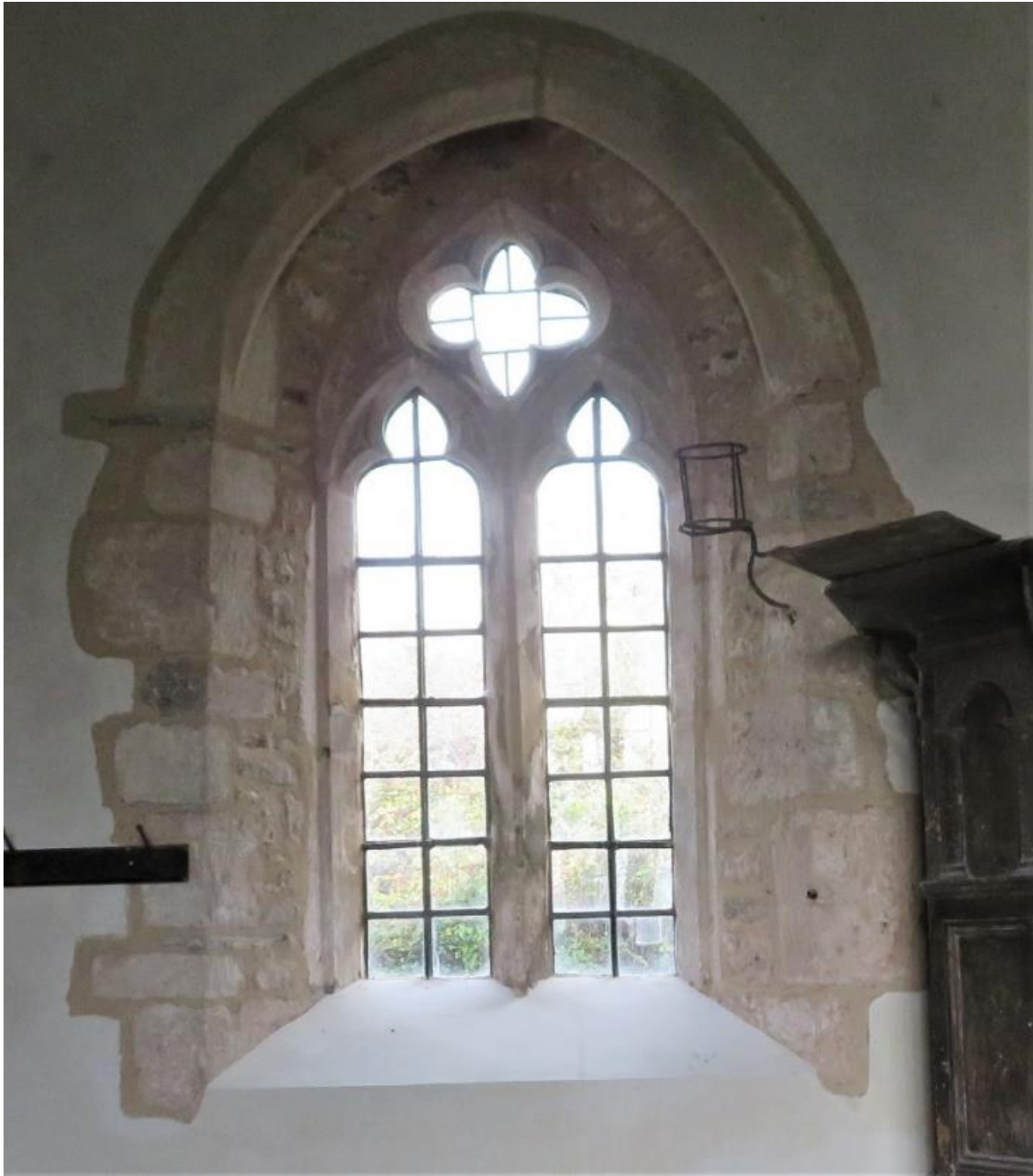
North side by pulpit. This two-light window with trefoil headed lights to each light is possibly 14 th century
