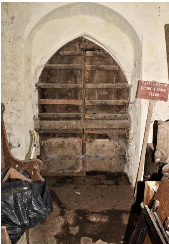
The west window and door.
