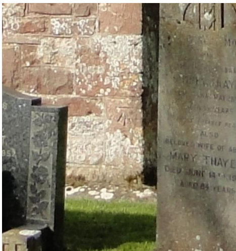
Fig 5: The Ordnance Survey mark.
