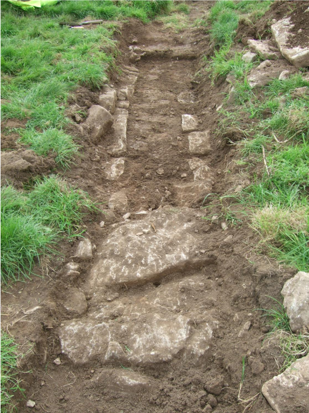
Fig 12: The gout with stone bridge
